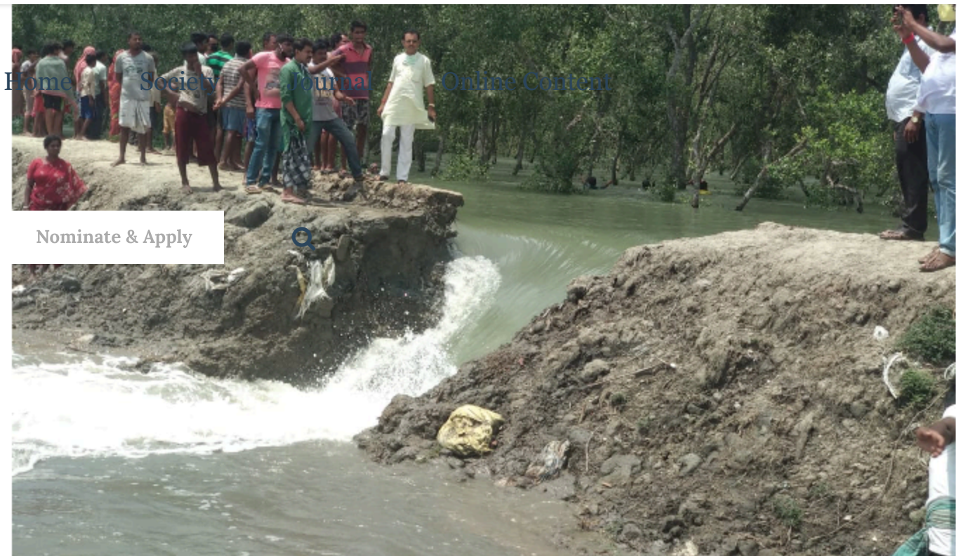
An earthen embankment breached by saline floodwaters following cyclone Amphan in Lahiripur village in the West Bengal Sundarbans. Photo by Ayan Ghosh. (India)
